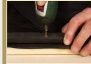
**16** Secure the floater frame using brass screws, being careful to select the correct length. Remove spacers.
